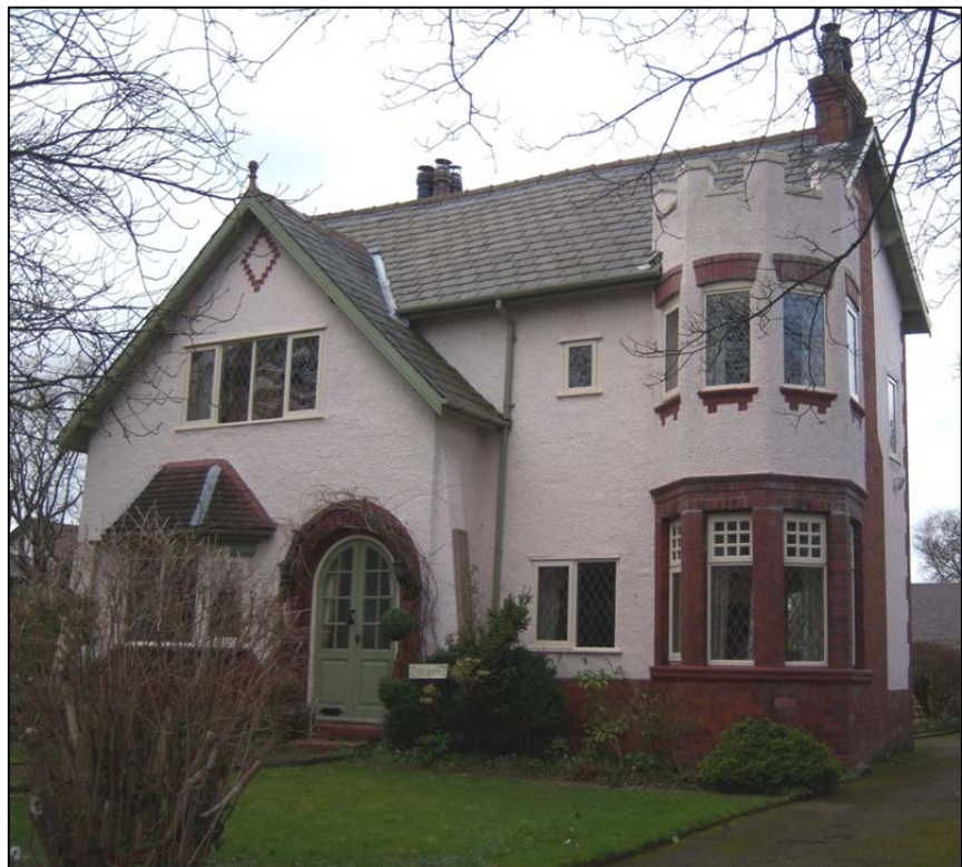
Another of the Edwardian properties - illustrating bespoke design but use of a common palette of materials and colours
